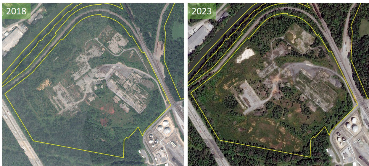
Figure 125. Canopy Loss in the Chattahoochee Brick Park
